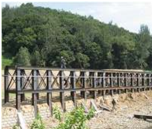
3. Completion bent installation
