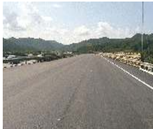
6. Temporary bridge completion
