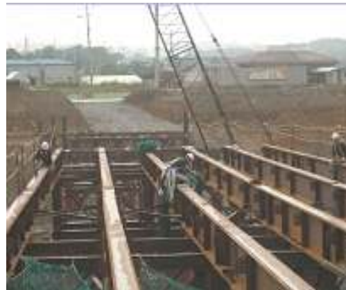
4. Girder and cross beam setting
